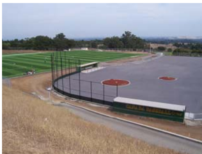
Baseball and soccer fields under renovation
