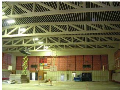
Renovation and Seismic Upgrade of Skyline Gymnasium
