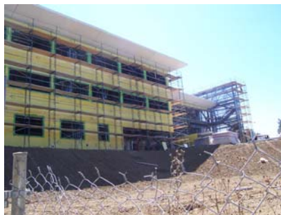
Integrated Science Center under construction
